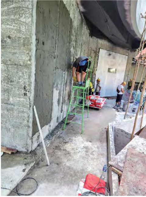
Plastering to external wall at frontage of Main Entrance
