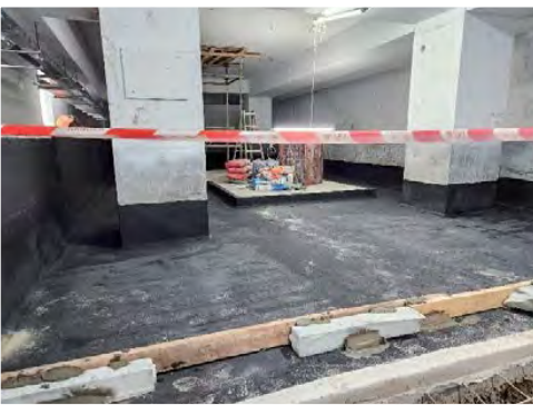
Getting ready for Water Tightness Test at the Filtration Plant Room
