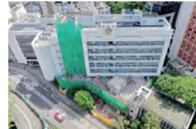
Commencement of Phase II of the School Enhancement Project
