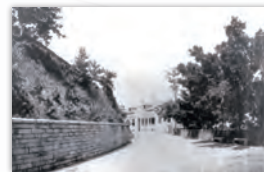
The buildings of St. Paul's College in Glenealy in 1888. (Credit: Public Records office, Government Records Service)
